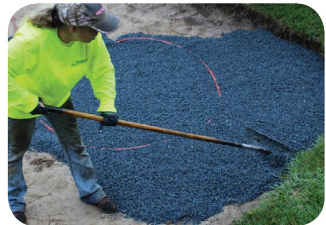
than fabric liners, and with more than three times the permeability of non-fabric liners, it drains rainwater from bunkers more quickly, keeping them playable."
